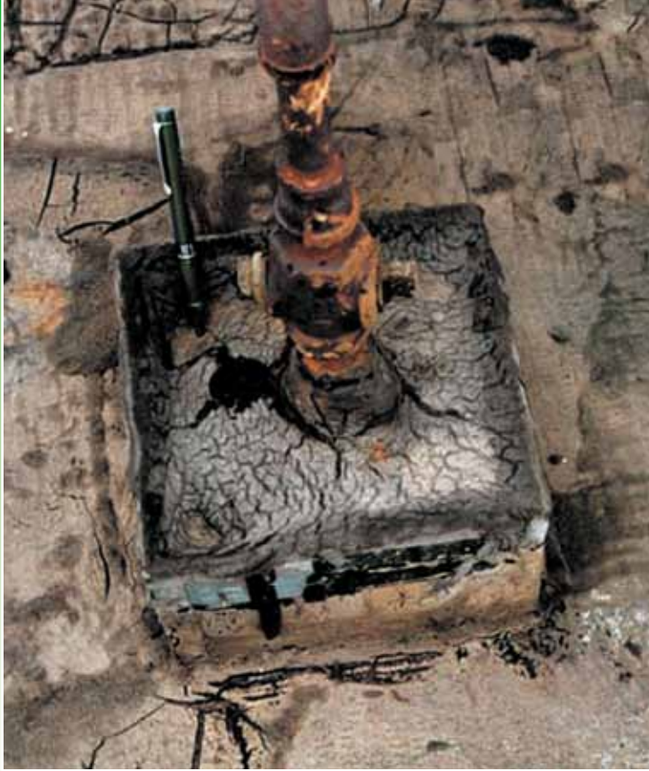
Cracked Pitchpan
